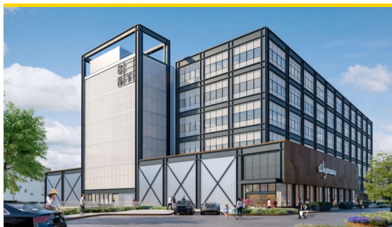
Admiral's Row at the Brooklyn Navy Yard will house the city's first Wegmans supermarket. Photo Credit: Brooklyn Navy Yard Development Corporation
